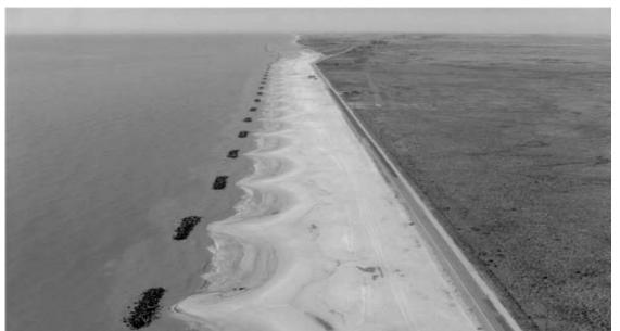
FIGURE 2. Holly Beach breakwater field, looking west from Louisiana towards Texas. The sub-aerial beach in this aerial photograph was constructed using sands buried in an offshore channel located about 3.5 miles offshore. Note the prominent salients forming in the lee of the emergent segmented breakwaters (Mann and Thomson, 2003).
